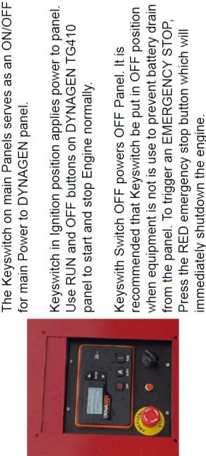
when equipment is not is use to prevent battery drain recommended that Keyswitch be put in OFF position
